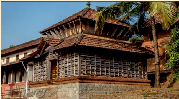
The Miyar house Entrance Block – 1856
